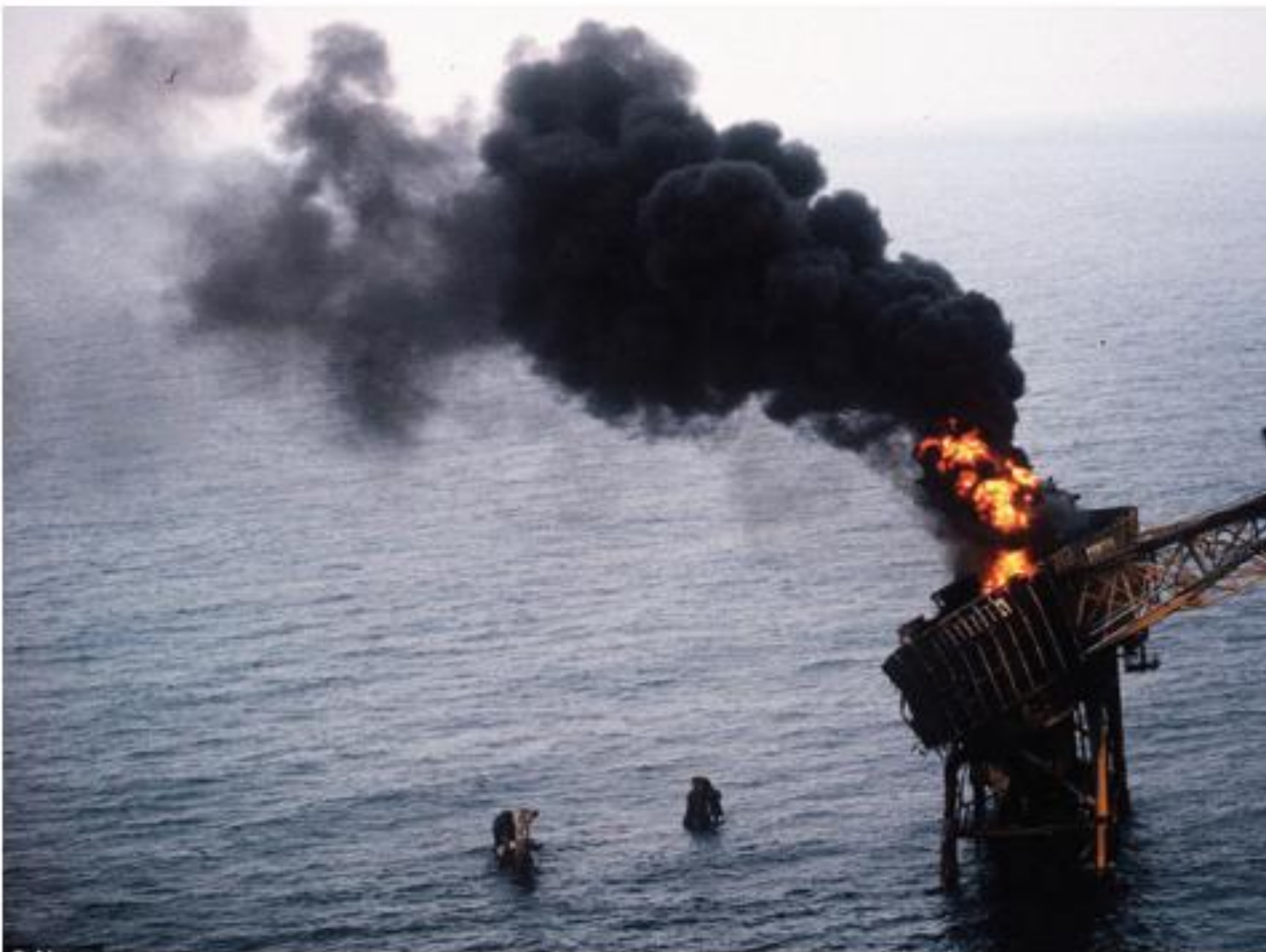
Figure 3. The remaining oil wells module continued to burn for weeks until famed firefighter, Red Adair, and his team extinguished the remains. Source: BBC.
